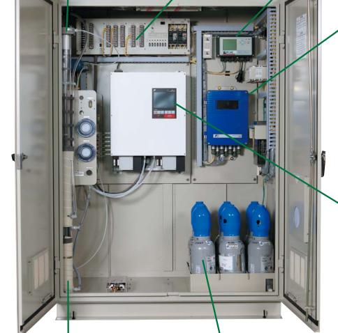
Gas conditioner to remove dust or drainage from flue gas
